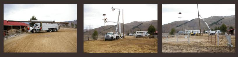
Before installing a web camera above the ospreys' nest that had been at Dunrovin Ranch for many years, Northwest Energy first had to move the nest off of one of its power poles. Electrical poles are not safe nesting platforms for ospreys as they can be easily electrocuted. Northwest Energy has an active stateside program to minimize the danger of its power lines to ospreys and other birds.
